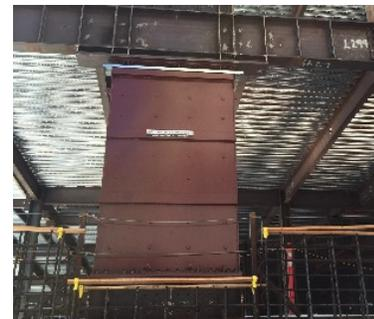
*Viscous wall dampers at the new California Pacific Medical Center (CPMC) Van Ness Campus hospital in San Francisco make the facility seismically sound.*
